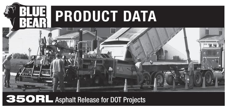
**350RL** is specially formulated as 100% biodegradable and is non-petroleum based. **350RL** prevents bonding of hot asphalt mixtures when applied to truck beds and other metal surfaces such as spreader and tools.
